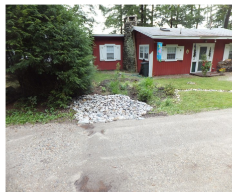
Riprap and rain garden installed on Hawk Road
